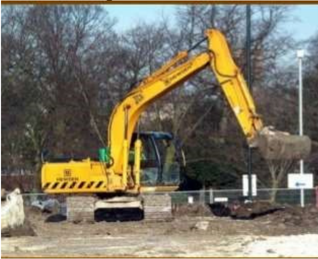
Picture taken at a construction by Chinese in Jubek state, Juba.
