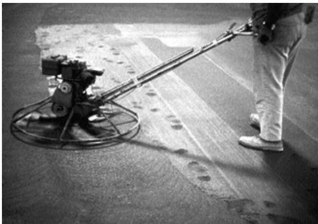
Power floating a screed
