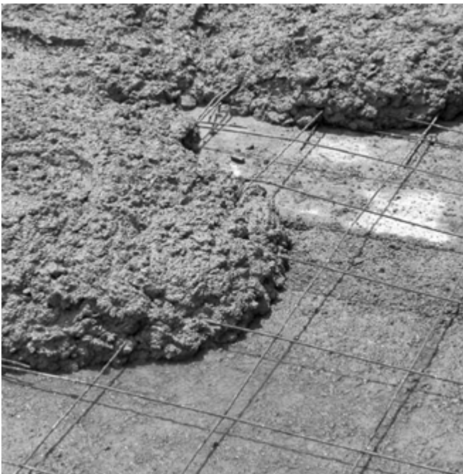
Concrete topping being placed on a precast floor.
